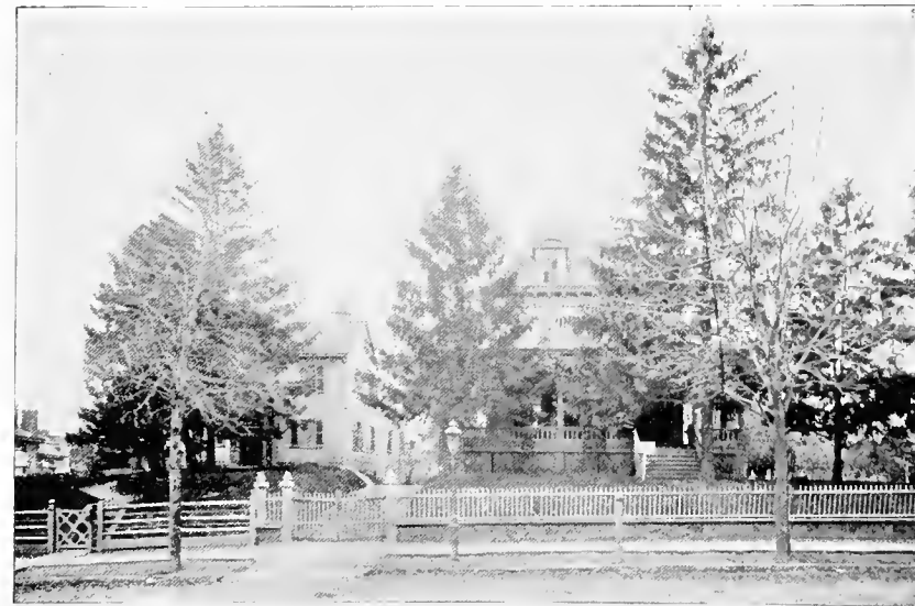
ST. LUKE'S HOME AND HOSPITAL—No. 153 Liberty Street.
